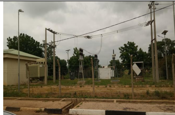
Figure 6: An existing power house in close proximity to the site
