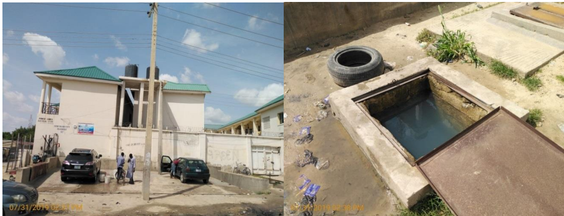
Plate 4.24: Water supply facilities observed in the community
