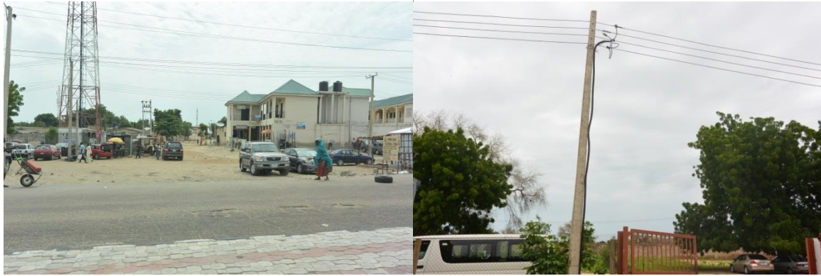
Plate 4.23: Electricity poles observed in community
