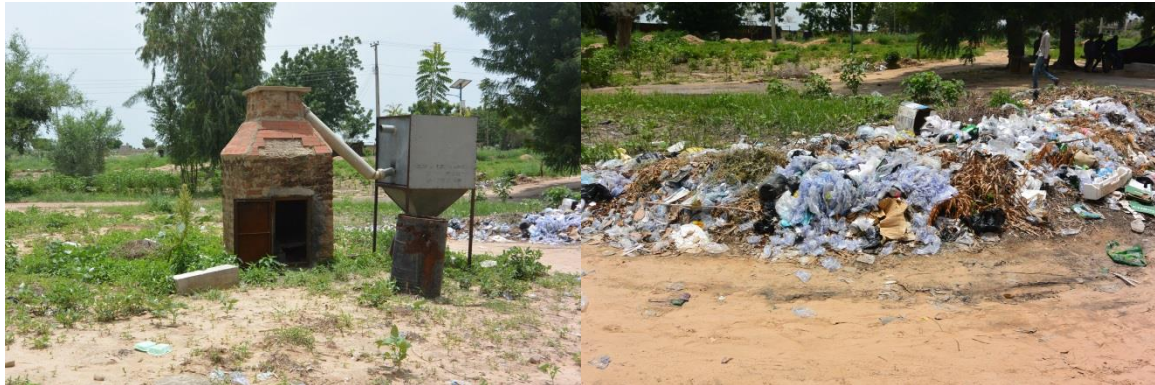
Plate 3.5: Waste management in UNIMAID (a) Incinerator (b) Open dumping
