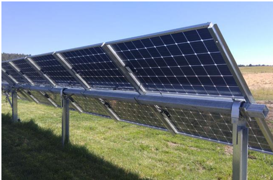
Figure 2.5: Bifacial Solar panels
