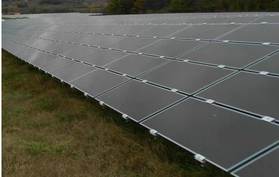
Figure 2.4: Typical appearance of Thin-Film CdTe panels
