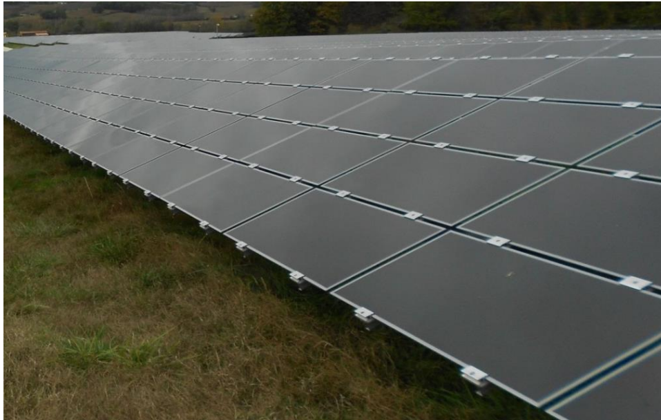
Figure 2.4: Typical appearance of Thin-Film CdTe panels
