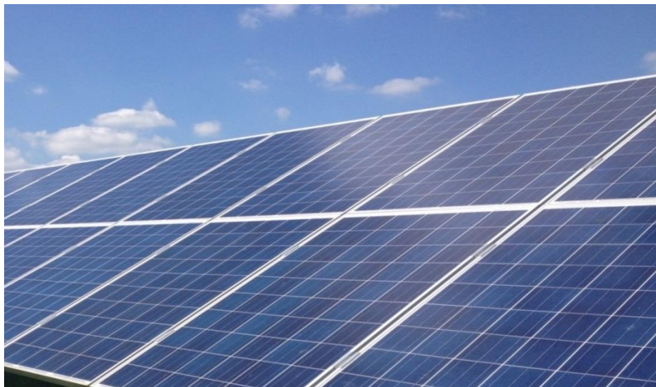
Figure 2.3: Typical Appearance of Polycrystalline Silicon PV panels
