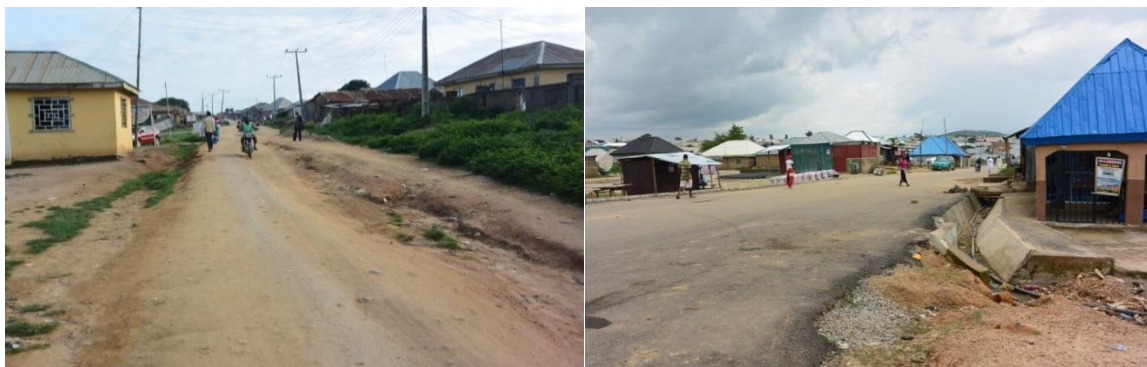
Plate 4.29: Road networks linking into the main community
