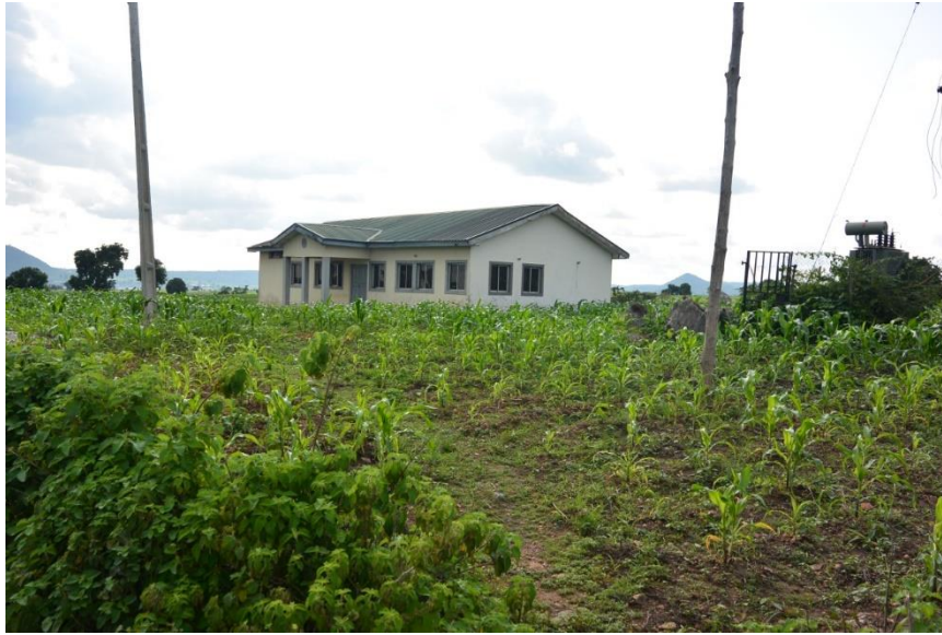
Plate 4.16: Unoccupied building observed on the site
