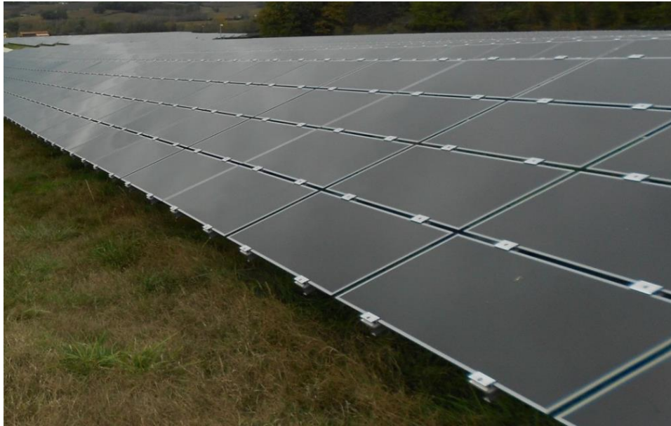
Figure 2.4: Typical appearance of Thin-Film CdTe panels
