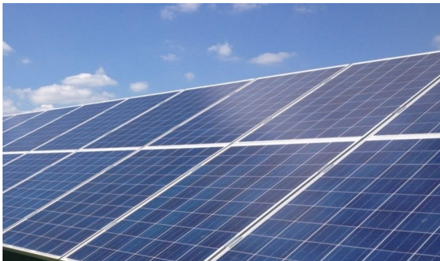
Figure 2.3: Typical Appearance of Polycrystalline Silicon PV panels
