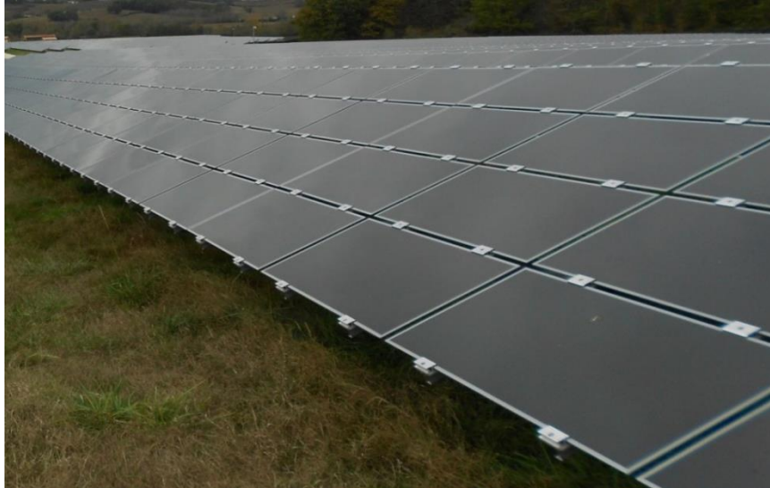
Figure 2.4: Typical appearance of Thin-Film CdTe panels
