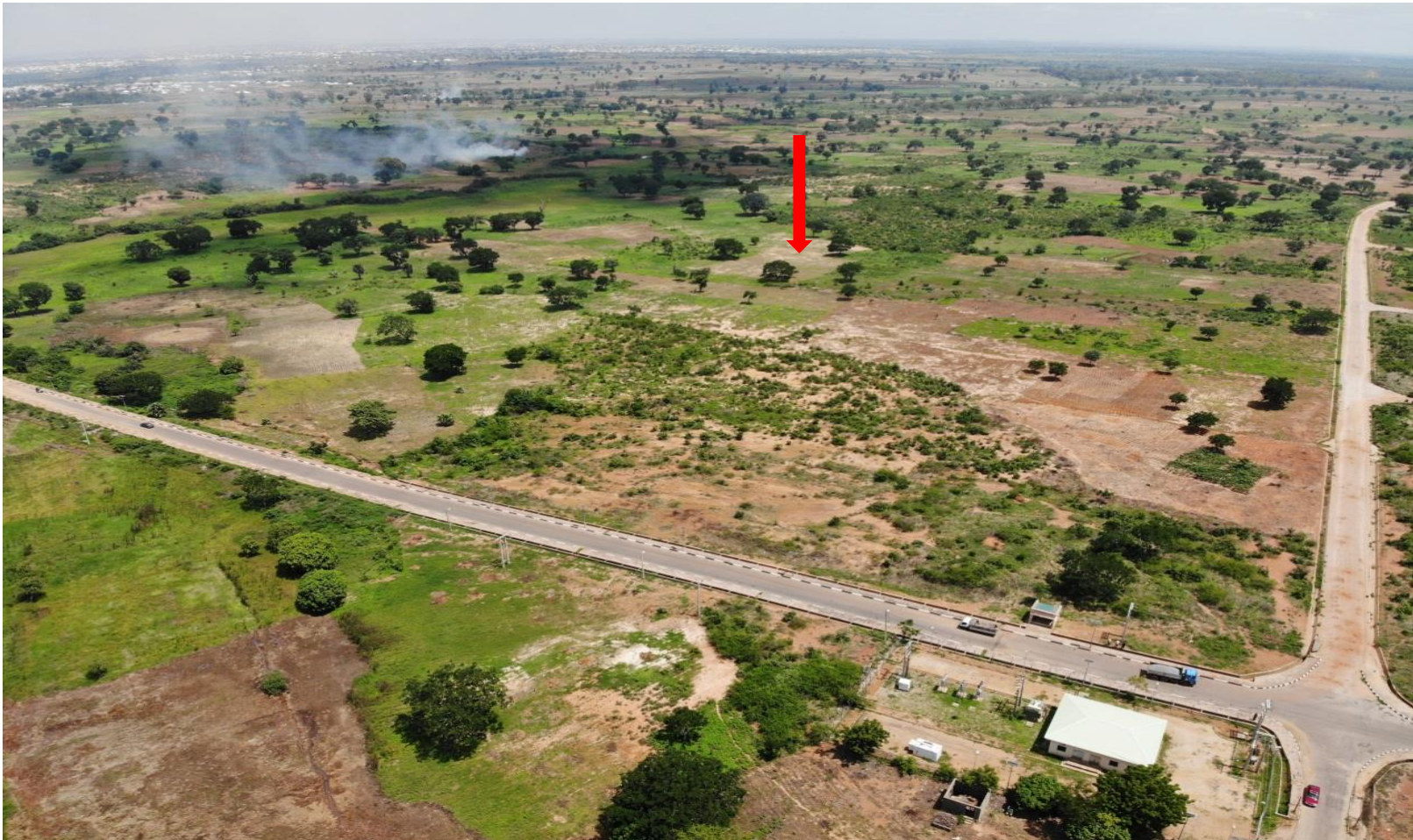
Plate 3.2: Aerial view of the Project site within NDA campus (shown with the red arrow)
