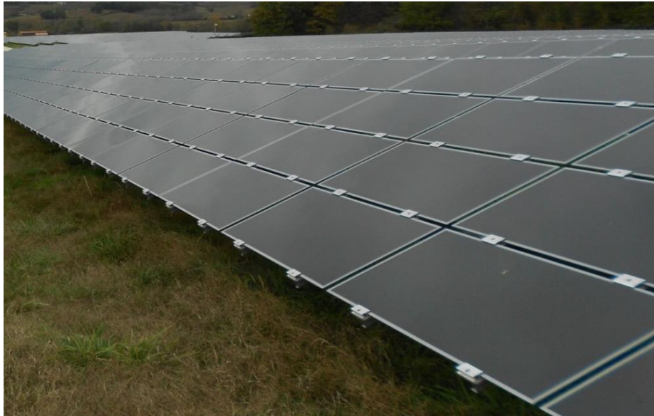
Figure 2.4: Typical appearance of Thin-Film CdTe panels
