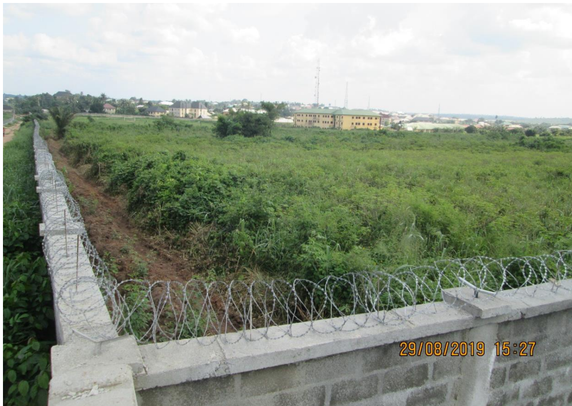
Plate 3.2: The boundary of the Proposed Project site at MOUAU Source: EnvAccord GIS, 2019
