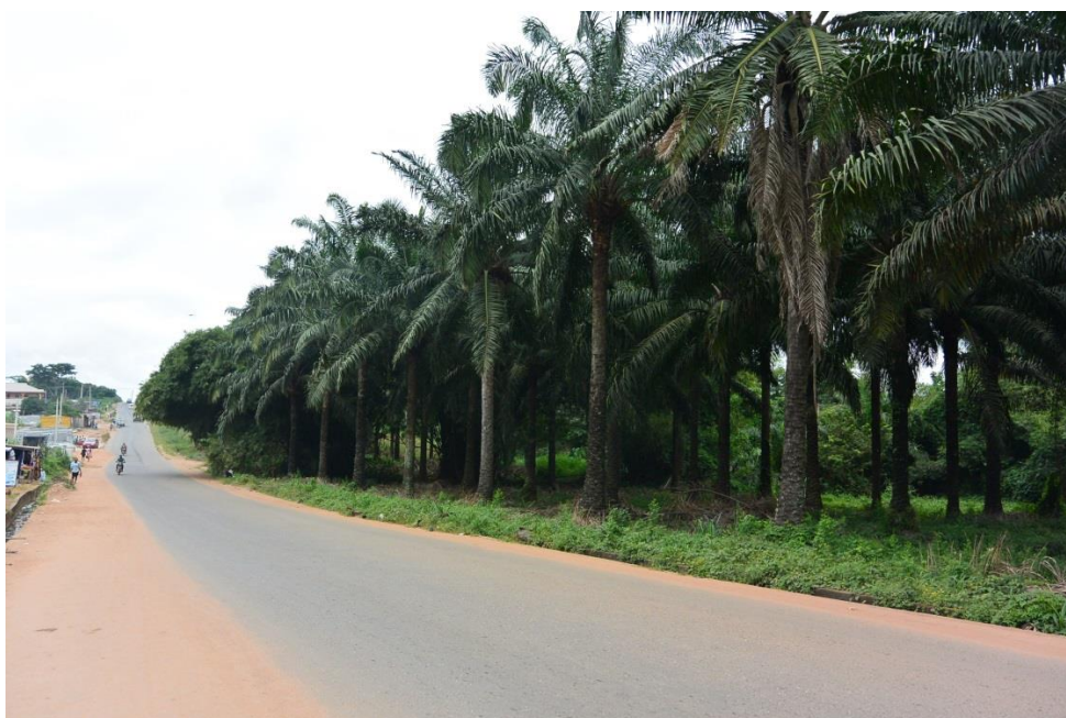
Plate 4.27: A view of the major road leading to the community
