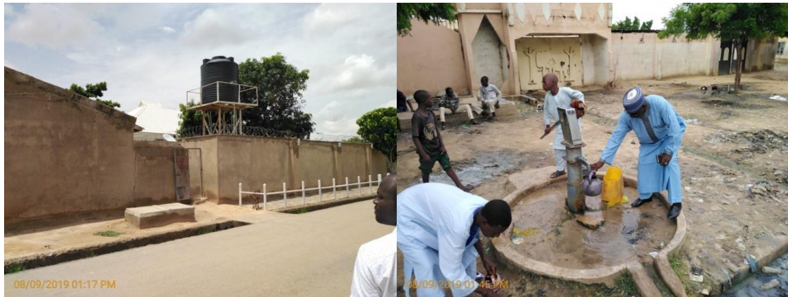
Plate 4.26: Water supply facilities within the community
