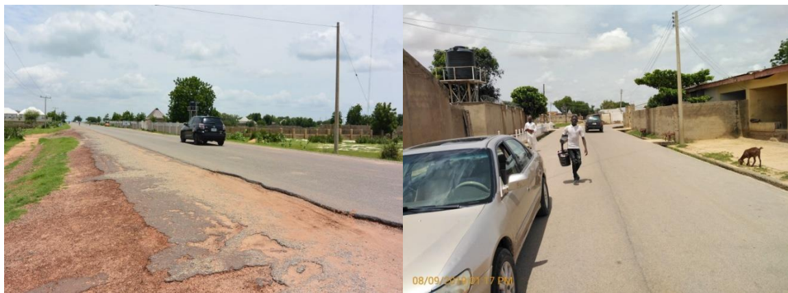
Plate 4.27: Road infrastructure within low-cost community
